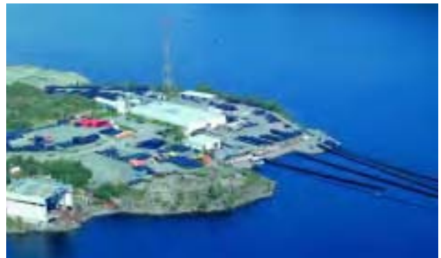
The Stathelle plant produces continuous pipe lengths directly onto the sea, where they are sealed and prepared for towing.
