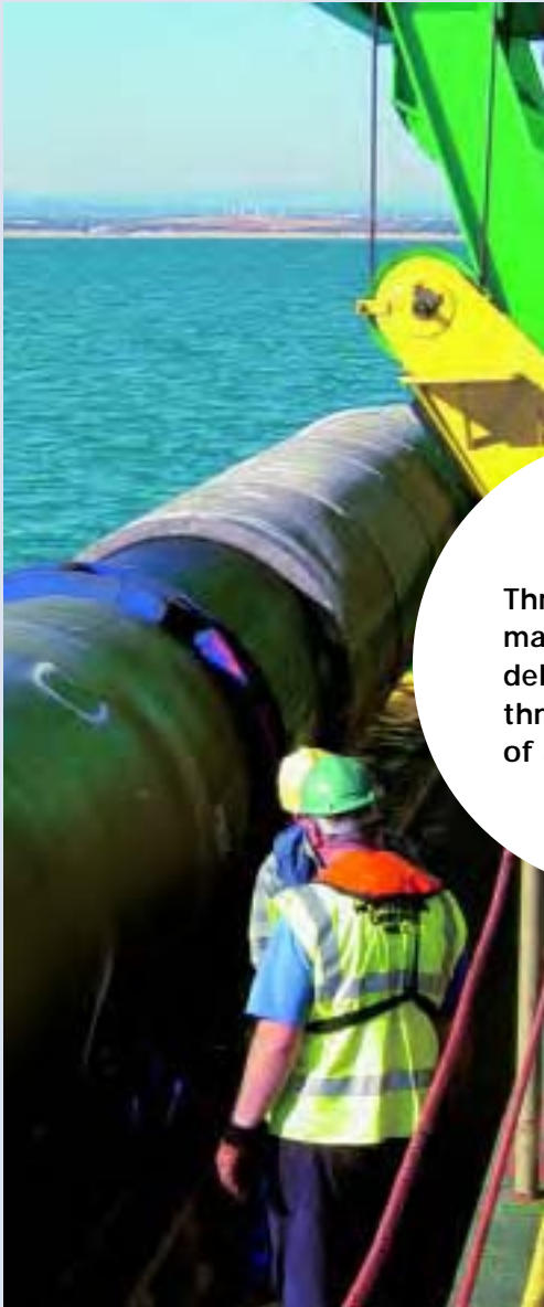
Connection of GRP coupling and submerging of the Ø 1600 mm PE outfall pipeline in Montpellier, France, 2003
