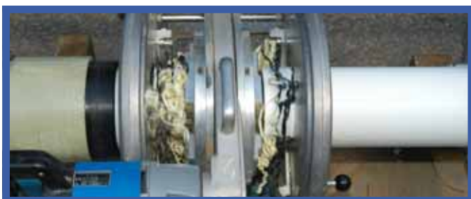
Photo 6: Trimming the pipe-ends
