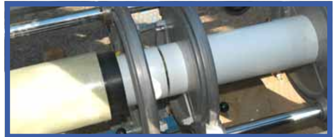
Photo 8: butt-welding of the pipe-ends.
