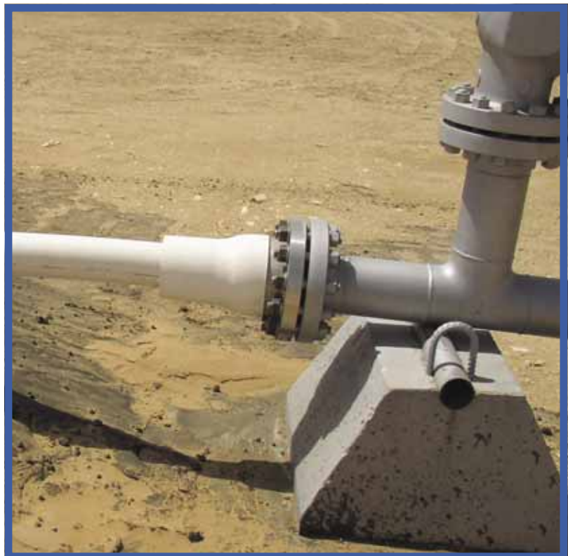
Photo 12: Installed Soluforce® end-fitting
