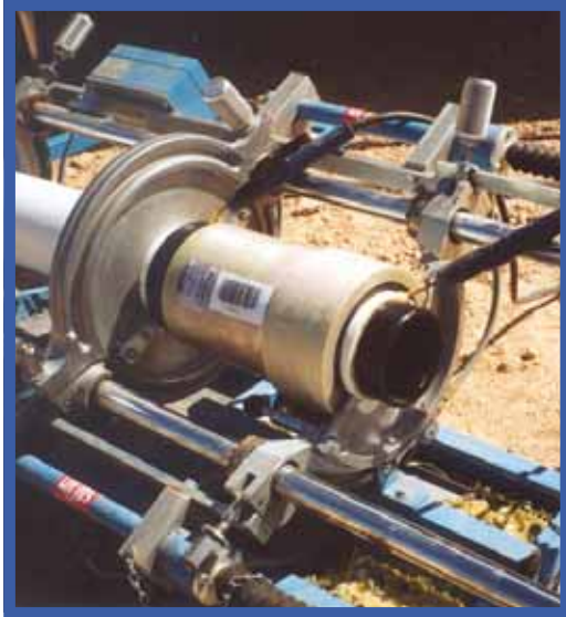
Photo 16: The actual welding of an end-fitting
