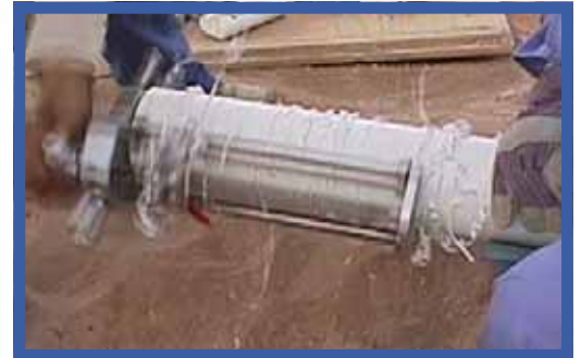
Photo 14: Scraping of the pipe outer surface
