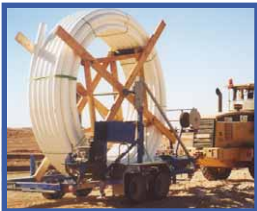
Photo 21: Soluforce® Coil loaded in the trailer and ready for uncoiling.
