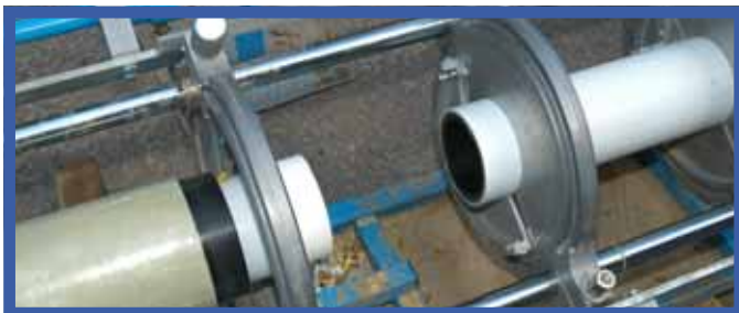
Photo 5: Pipe-ends loaded in fusion frame
