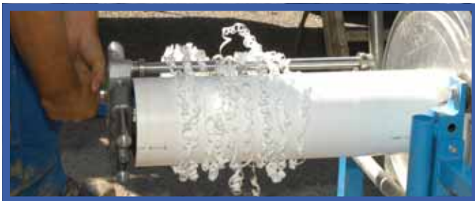
Photo 4: Scraping the pipe cover layer
