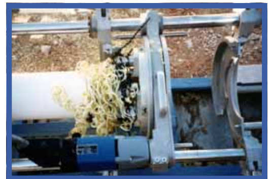
Photo 15: End-fitting trimming in progress
