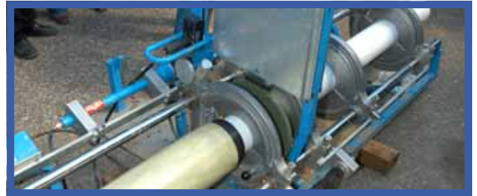
Photo 7: Heating the liner-pipe ends by means of the heating-plate
