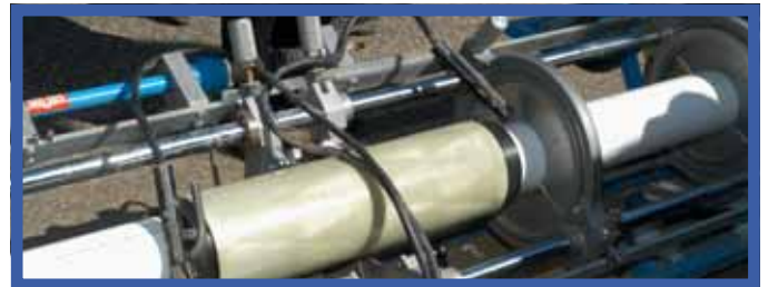
Photo 9: In-line coupler electrofusion sleeve centrally placed over the pipe-ends and connected
