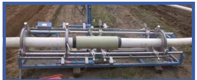
Photo 10: After cooling the in-line connection is ready
