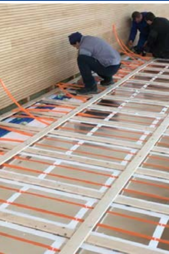
Pipelife underfloor heating installation for Zabok Sports Hall, Croatia.
