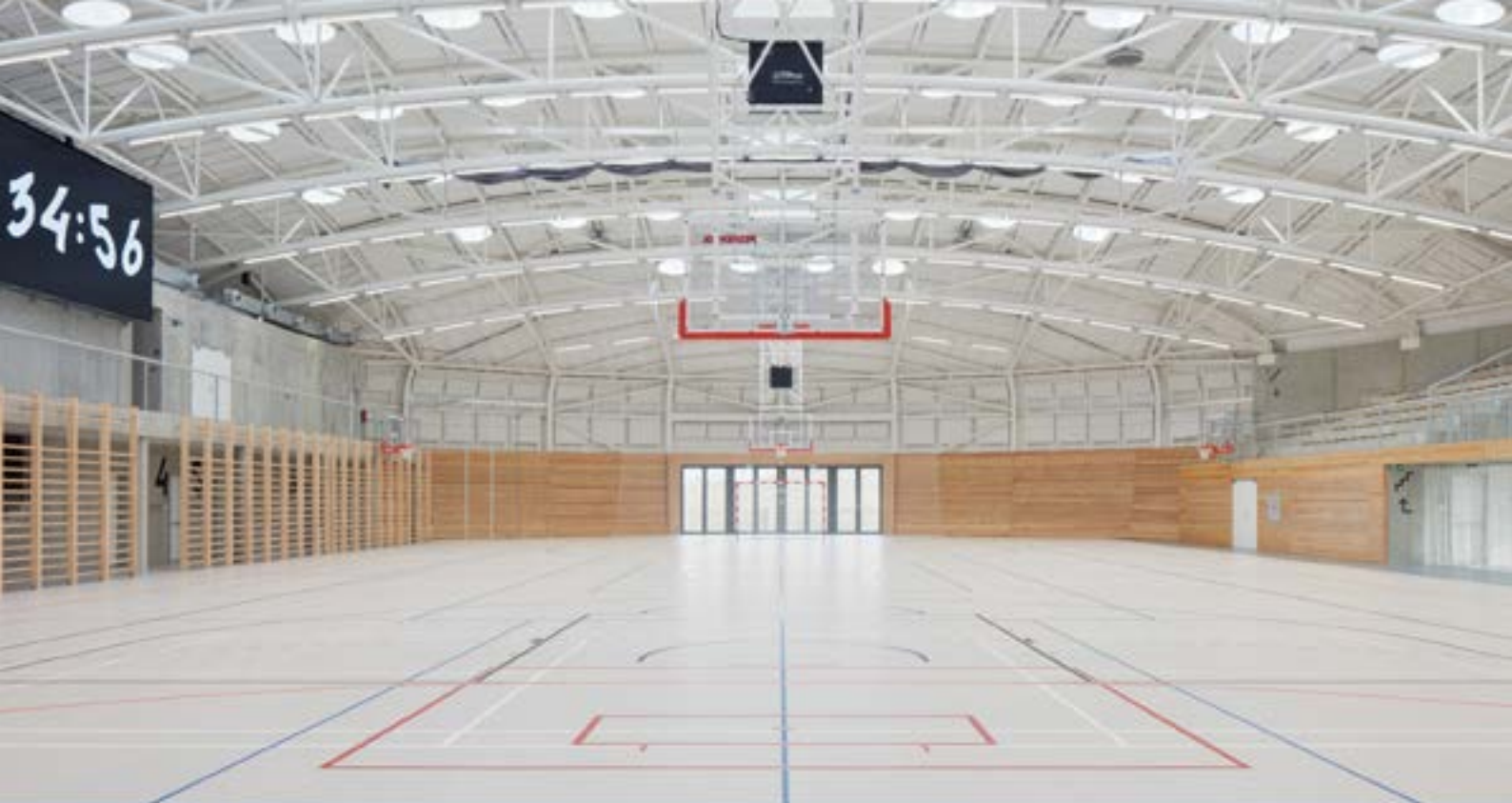
Pipeline underfloor heating installation for Dolní Břežany sports hall, Czechia.*
