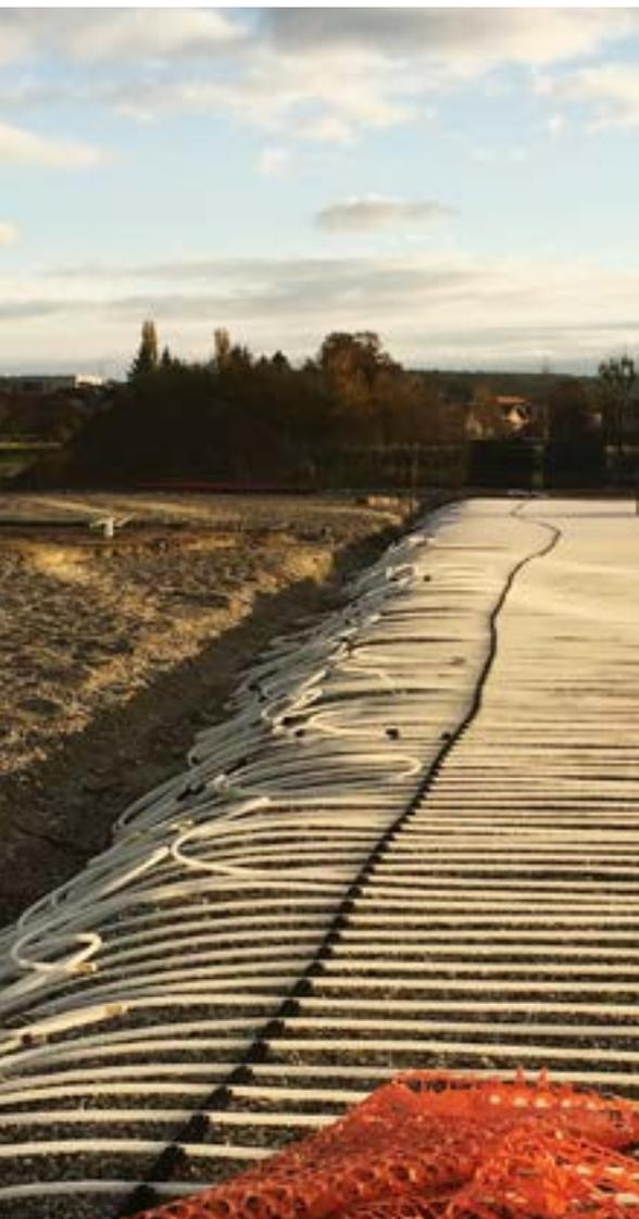
Compare how pipe spacing and pipe diameter variations with screed flooring affect the supply/return temperature of the heating fluid, and as a result, the efficiency of the hydronic radiant system.
