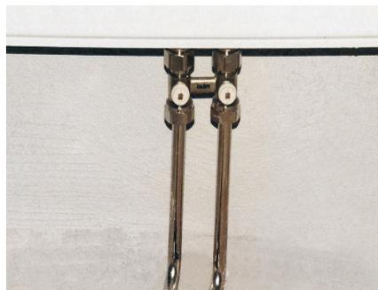
Assembly with radiator connecting elbow fittings
