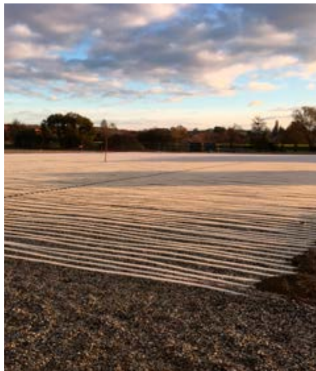
Undersoil heating pipes being installed at Terme Vivat Complex in Slovenia.
