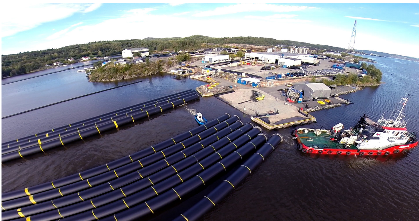
Pipelife Norge Stathelle plant
