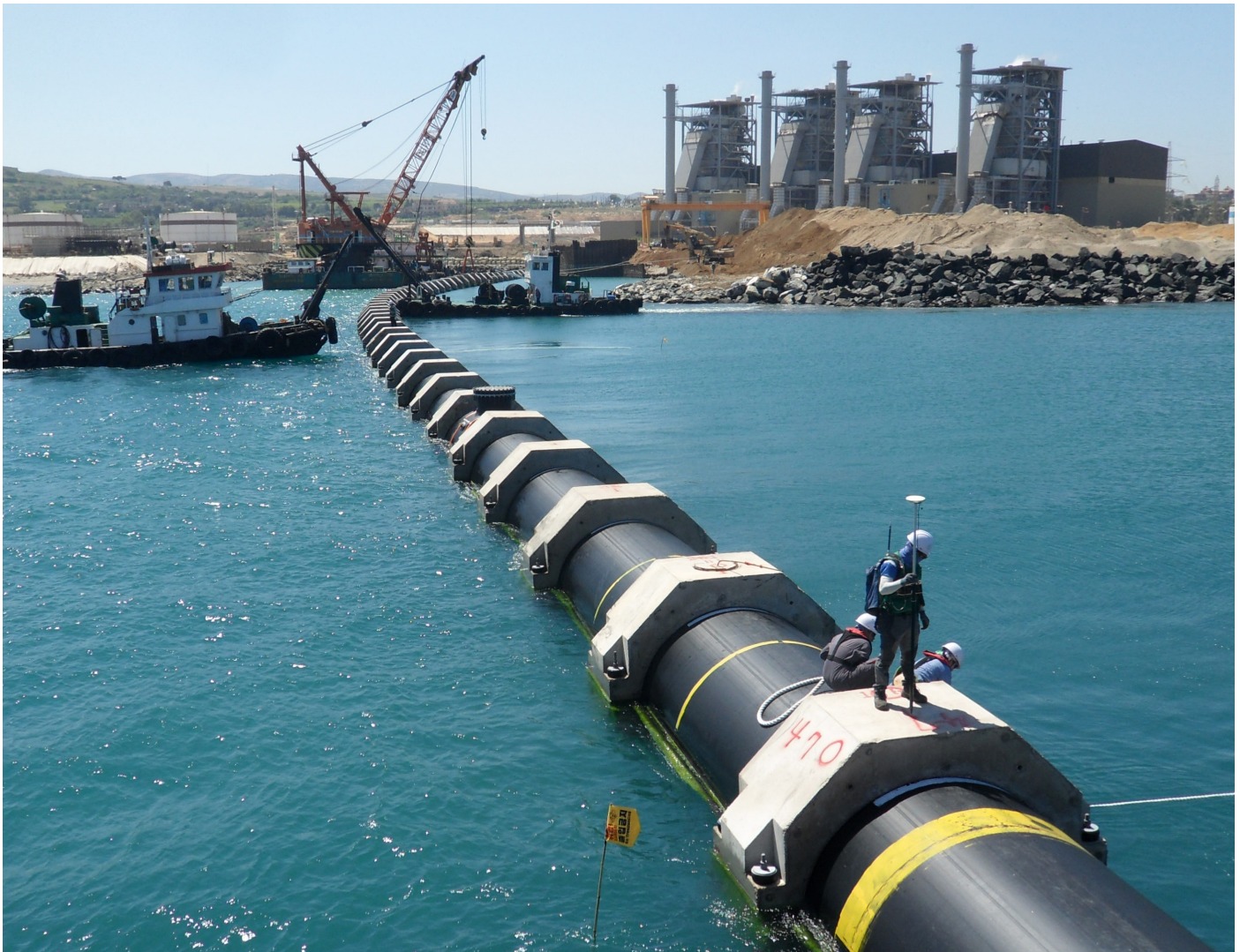
Beginning of submerging of OD2500 mm SDR26 pipe
