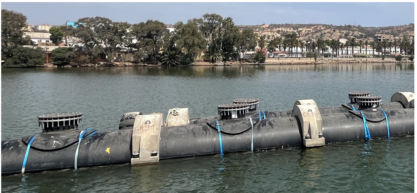
Completed saddle fittings with temporary blank flanges ready for installation
