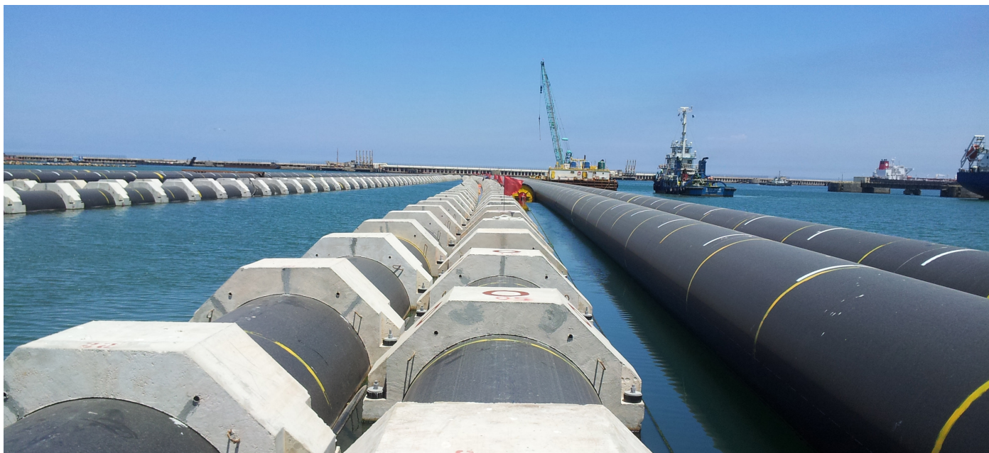
Typical pipe collar weighting for marine installation
